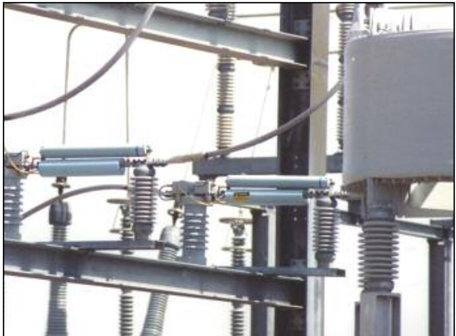
▲ Structure mounted 38kV, 1200A CLiPs in a reactor bypass application.
