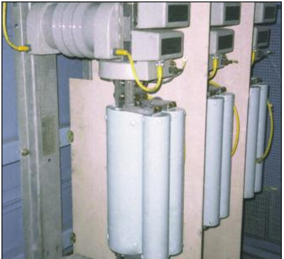
▲ 5.5kV, 1200A CLiPs mounted in an enclosure.
